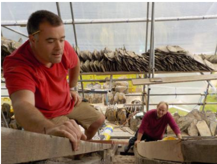
Timber repair in progress
